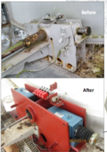
Elevation safety components refurbished
