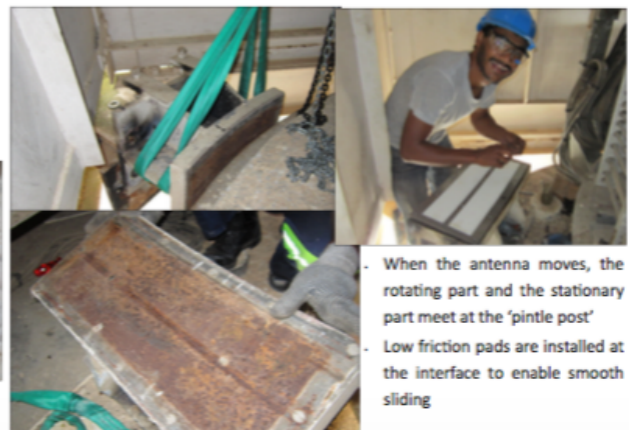
Replacement of pintle pads
