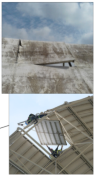
Surface panels repaired and refurbished
