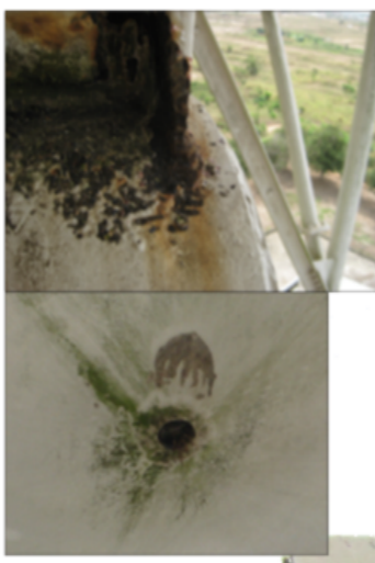
Rust, algae removal and painting
