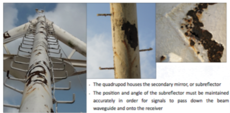
Subreflector support ("quadrupod") legs replaced
